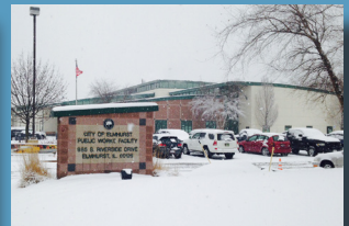
PUBLIC WORKS FACILITY 985 S. Riverside Dr. (630) 530-3038
